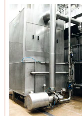
Irrigation cooler for ice water and brine refrigeration cycle with filter systems.
